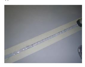
The joint faces should be protected with masking tape to facilitate tooling.
